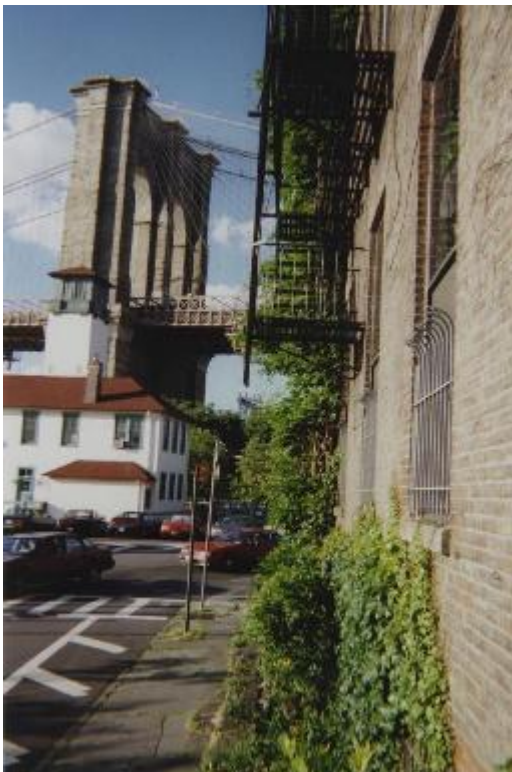
Figure 4. Apartment Building Showing Proximity of Bridge
